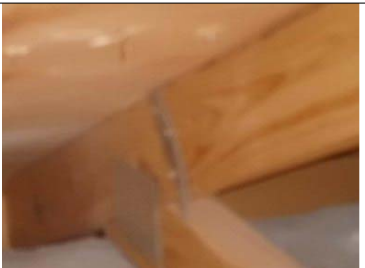
Roof to wall attachment
