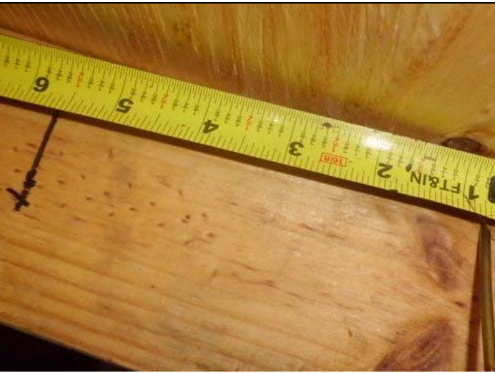
Roof deck attachment
